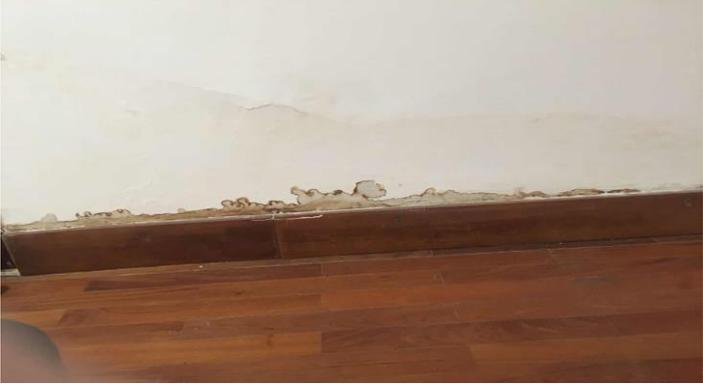
A photograph showing a wooden skirting board at the base of a wall. The board is broken and the top edge is crumbling, with some white material visible underneath. The floor is made of dark wood.               |
