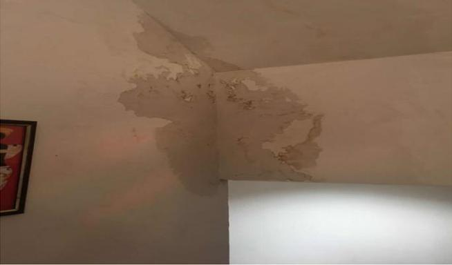
A photograph showing a corner of a room where the wall has significant water damage. The paint is peeling and the surface is stained with brownish water marks. A small framed picture is visible on the left wall. |
