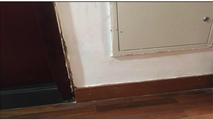
A photograph showing a door frame that is severely damaged and partially missing, revealing the interior structure. A wooden floor and a white cabinet are also visible. |
